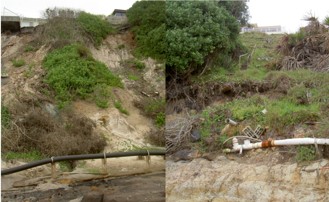
Figure 2: A photo of the original sub-horizontal drainage scheme installed in 2001 destroyed by wave erosion and embankment slippage
