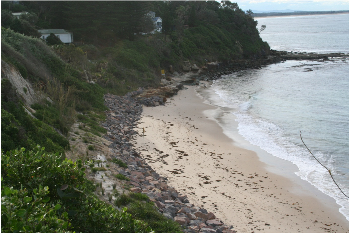
Figure 9: A photo of the completed TDS looking north (June 2013)
