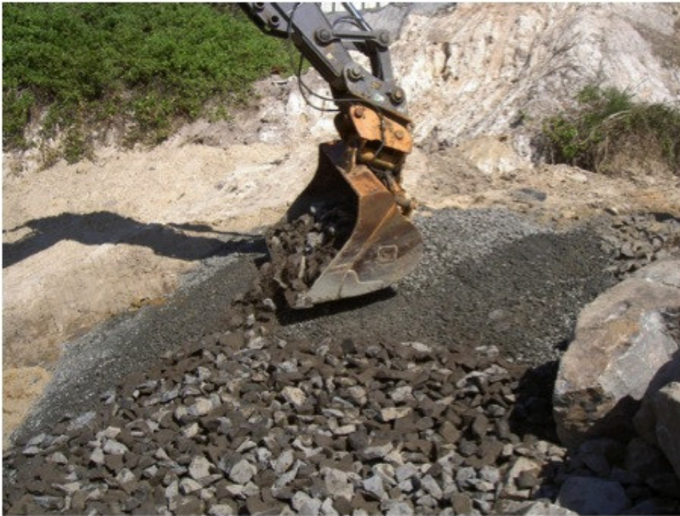
Figure 4: A photo of the placement of the graded filter layers (July 2011)
