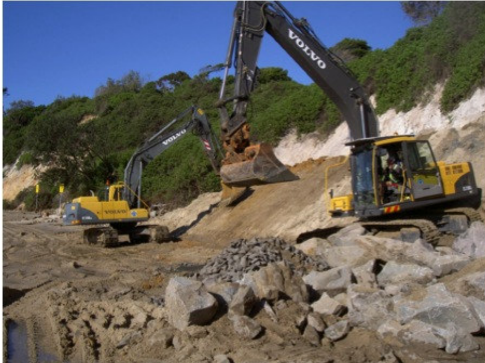
Figure 5: A photo of the 20T excavators working in tandem on the beach in CTH (July 2011)
