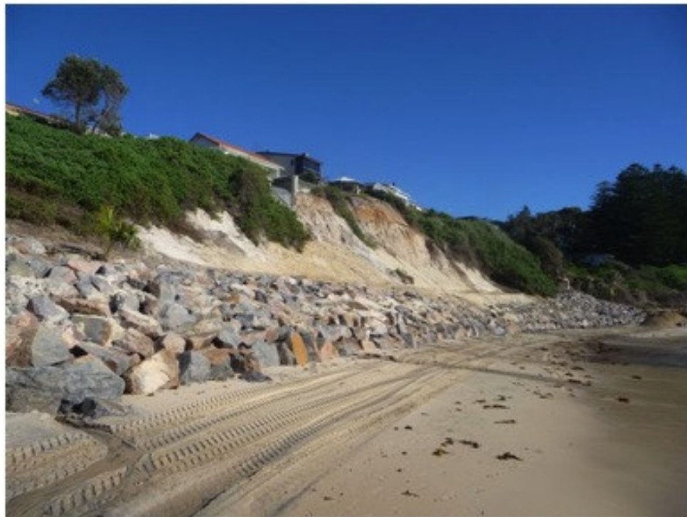
Figure 8: A photo of the completed TDS from beach level looking north (September 2011)
