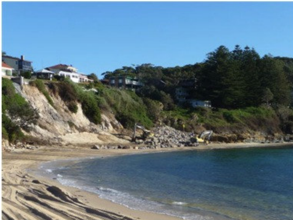
Figure 6: A progress photo of the construction of the TDS at north end of CTH (July 2011)
