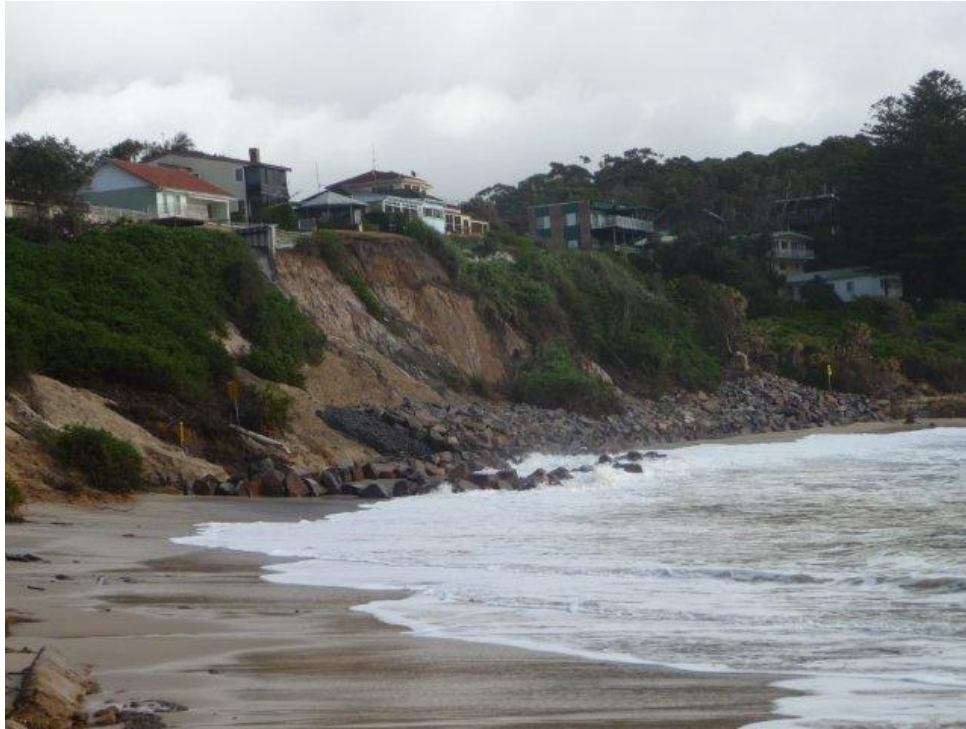
Figure 7: A progress photo taken during one of the few days lost to adverse weather. Note the armour rock used to form a temporary barrier to protect the work (July 2011)
